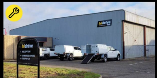
Adelaide Showroom & Installation 6 Wirriga St, Regency Park SA 5010
