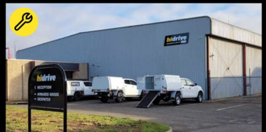
Adelaide Showroom & Installation 6 Worriga St, Regency Park SA 5010
